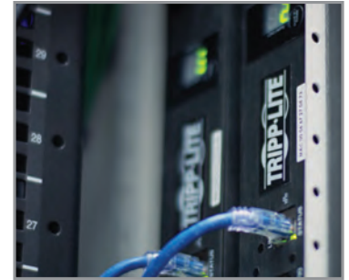
Tripp Lite’s WEBCARDLX provides remote management of compatible UPS systems and PDUs.
