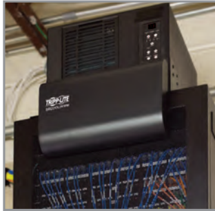
Tripp Lite’s SRCOOL2KWM provides 2,000 BTU of air conditioning for wall-mount rack enclosures.
